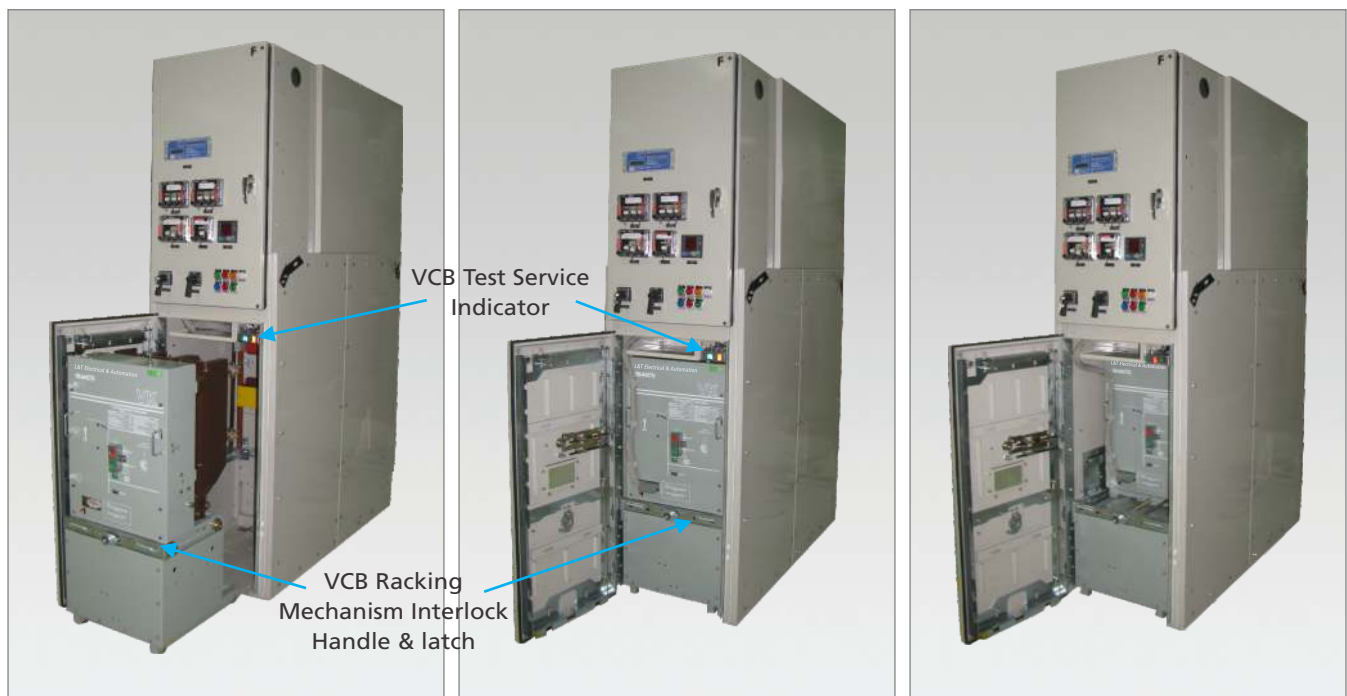
Figure 5.1 A - VCB in Disconnected
